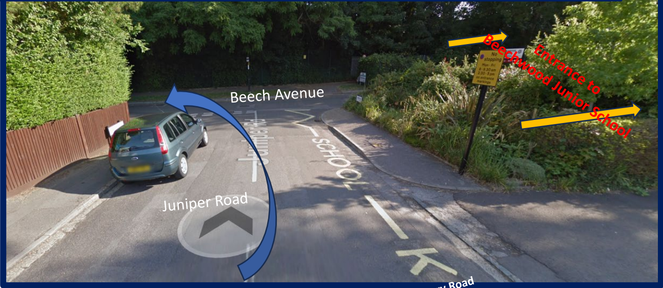
Approach Road - Juniper Road into Beech Ave by Beechwood Junior School
